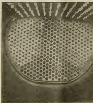
FIRE BOX END OF LOCOMOTIVE BOILER TUBES PARTIALLY WELDED. LIGHT AREAS SHOW WELDED TUBES AND DARK AREA SHOWS TUBES READY FOR WELDING.
